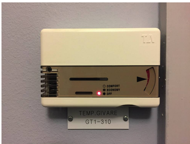
Figure 13. The BMS thermostat in the office room
